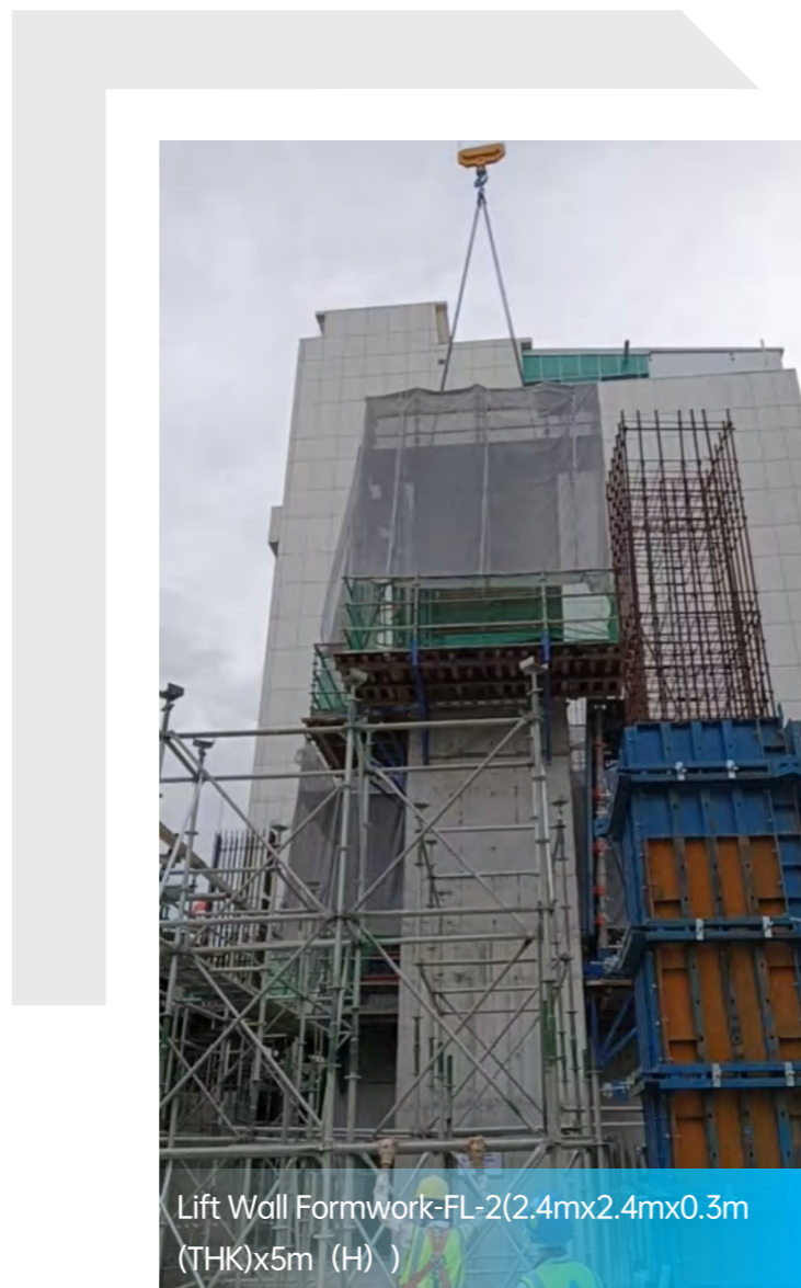
Lift Wall Formwork-FL-1(6.7mx3.mx0.3m(THK)x5m (H) )&FL-2(2.4mx2.4mx0.3m(THK)x5m (H) )
