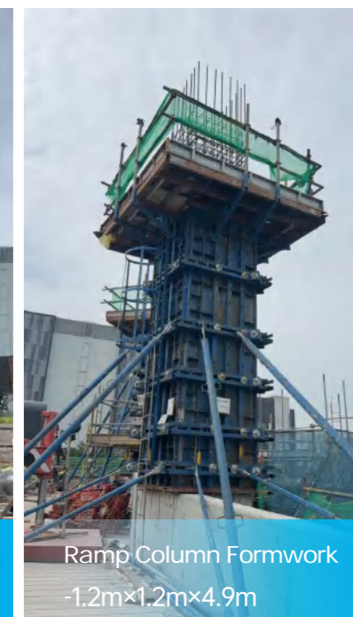
Ramp Column Formwork -1.6×1.6×4.3m
